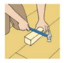
Tap the new board in place using a Tapping Block, beginning on the long side.
